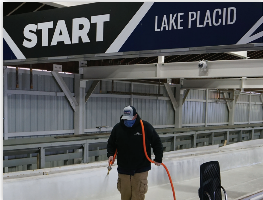
Ricky Fredrick of the Lake Placid ice crew resurfaces the track using the Tundra hose.
